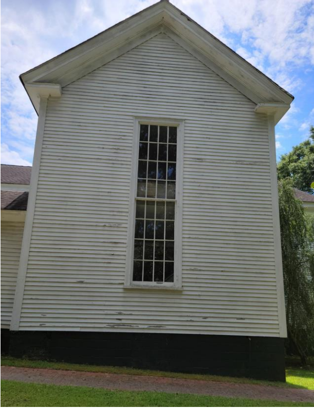
North Transept View
