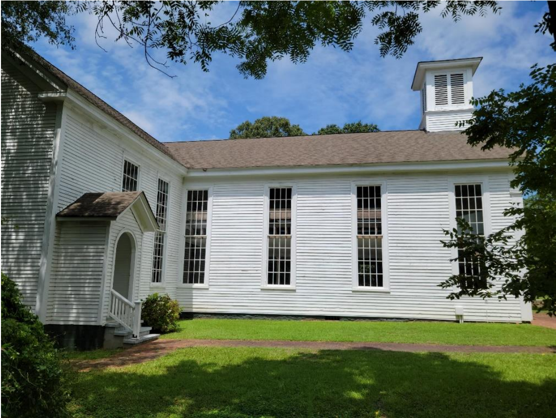
South Nave View
