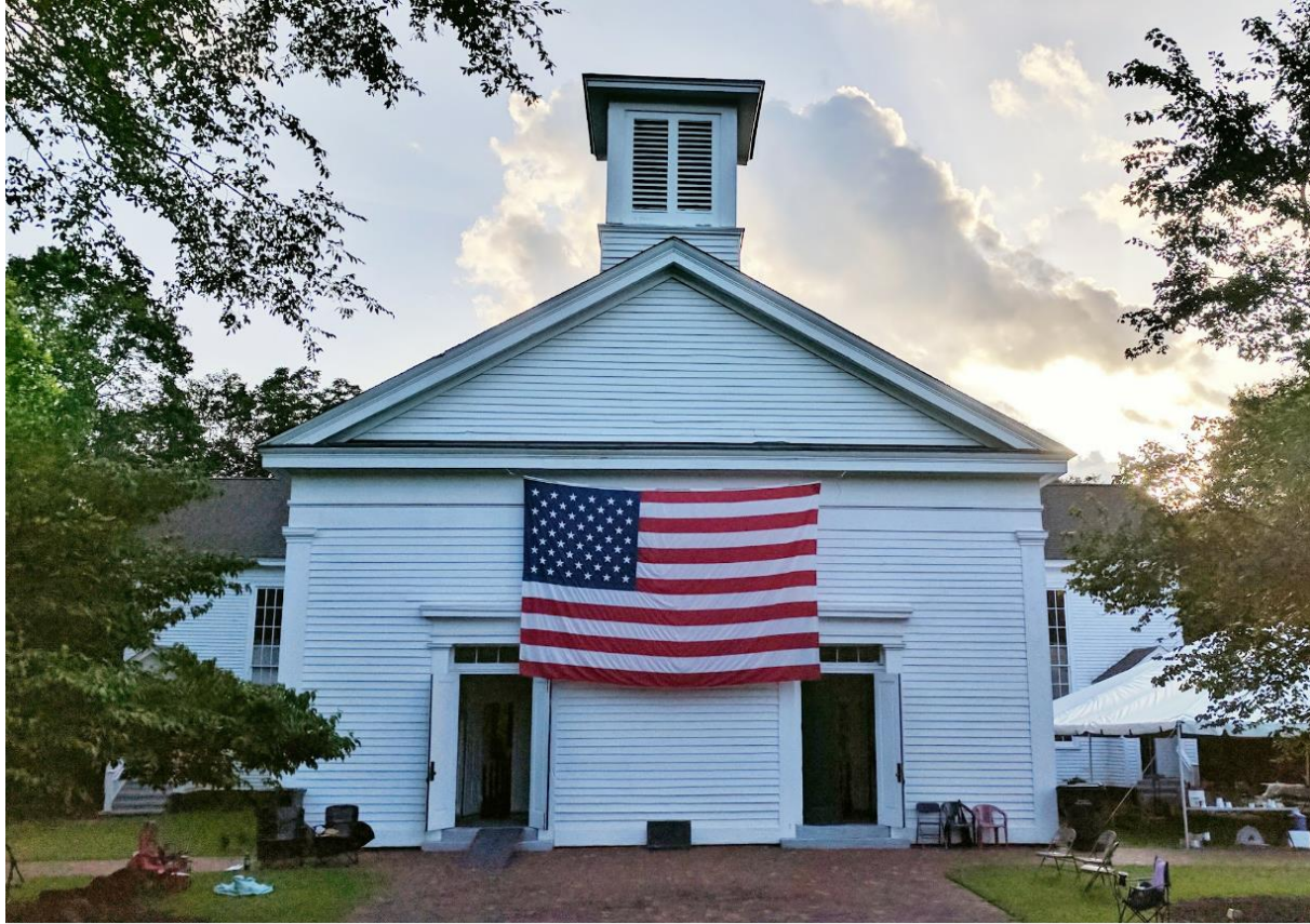
East Front View
