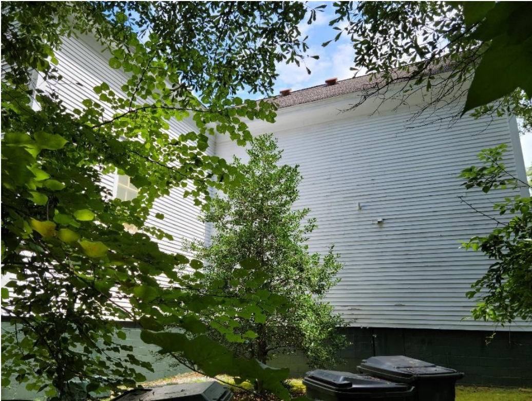
West Rear and South Transept View – Tree will be removed as necessary by City Staff
