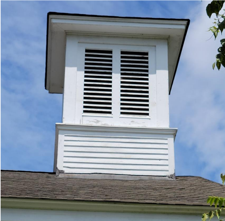
Bell Tower Detail
