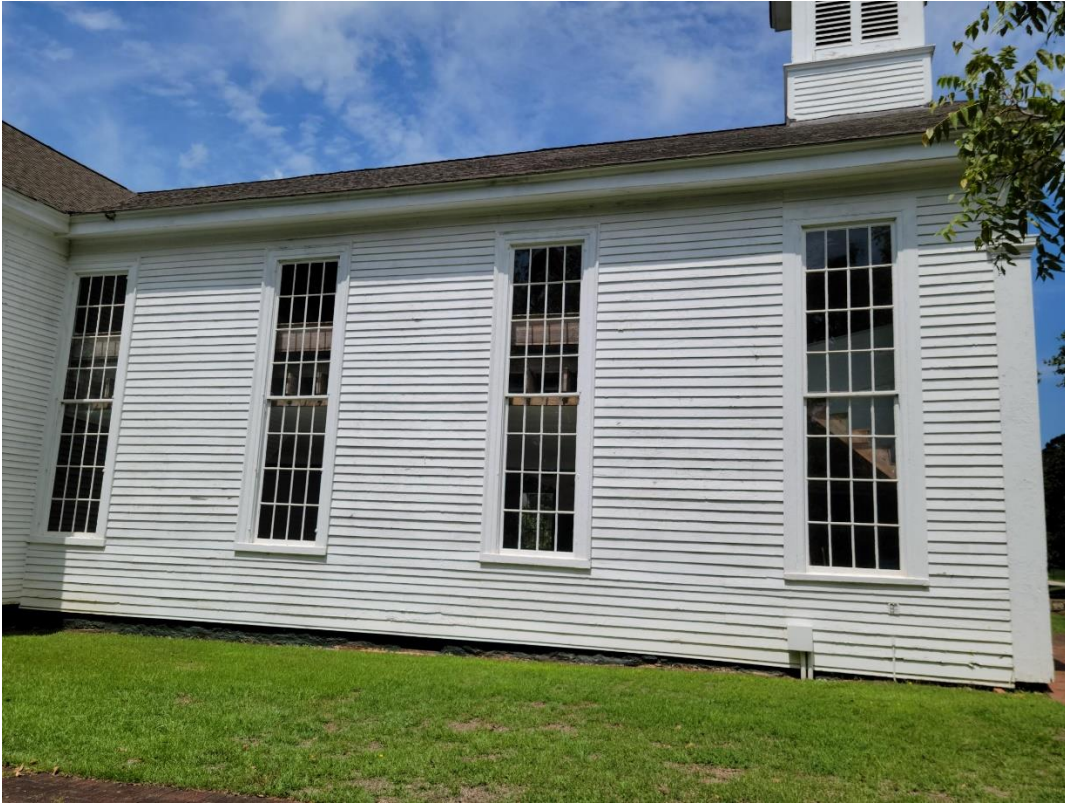
South Nave View
