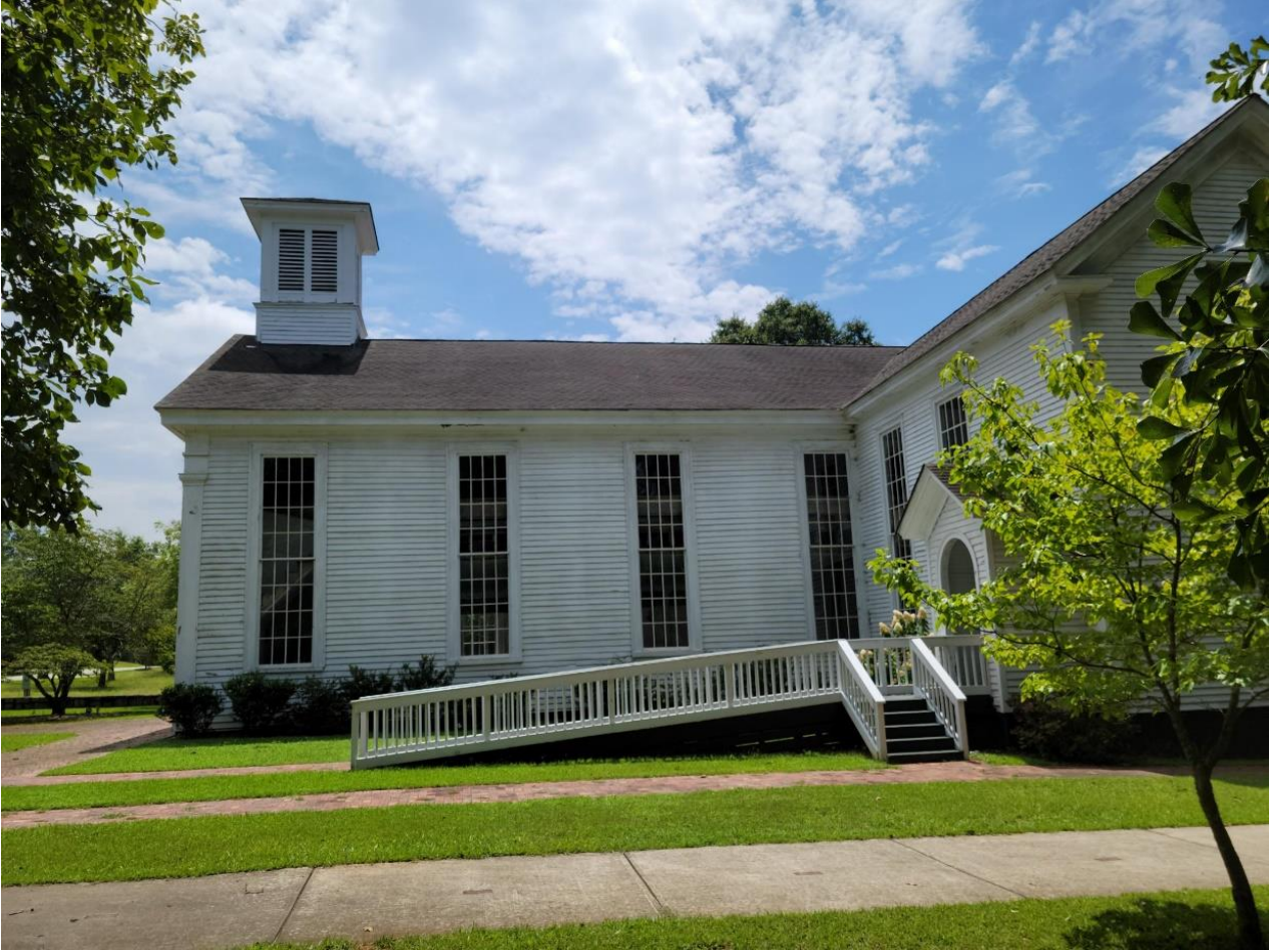
North Nave View
