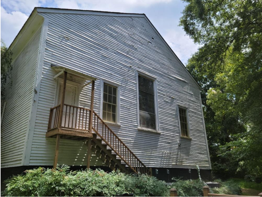
West Rear Side View
